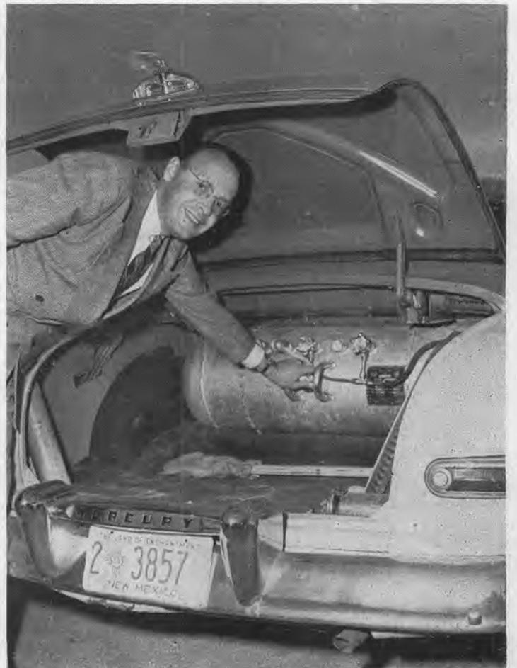
G. C. "Corry" McDonald explains the operation of the butane fuel system he has had installed in his car. Corry's car will operate on either butane or gasoline through use of a dual carburetor. Fuel costs less if butane is used, but there are several drawbacks to its use. For Corry's account of the advantages and disadvantages read the accompanying story.
