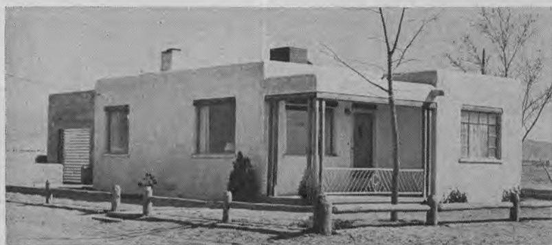
Here is the home of Mr. and Mrs. Harold Cripe which they built with their own hands. They are still working on the home and are about to complete the new garage seen at the left.
