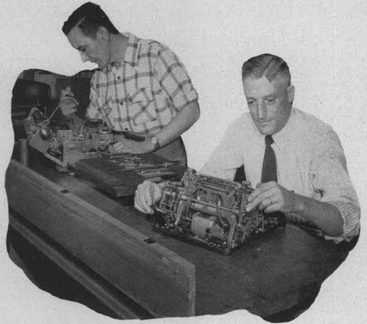
COMPLETE OVERHAULS are performed in the shop at the rate of an average of two a day. Here Felix Padilla (left) works on a typewriter while Bill Olheiser overhauls a calculator.
