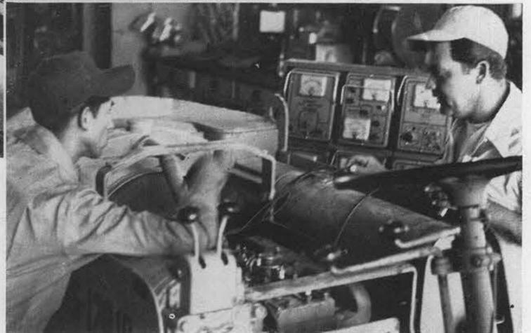
**MOTOR ANALYZER** leads are run into a fork lift by Charles Garcia as the boss, "Luke" Luker, stops by. If there's anything wrong with the lift's motor or electrical system the analyzer test gauges will find it.
