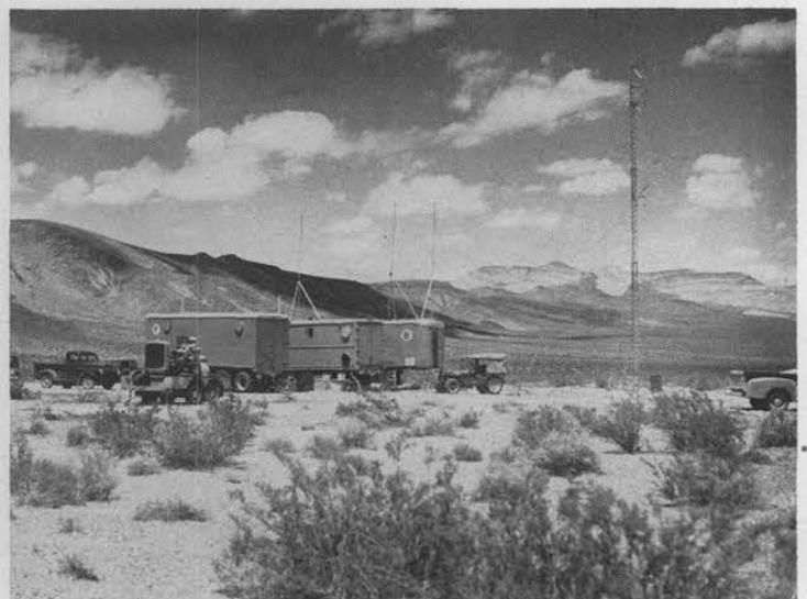
HUDDLED in the sage clumps of the Nevada desert are three Project Outcast trailers. Shown here are two telemetering labs and a mobile photo processing laboratory for on-the-spot development of field test results and photographic material.
