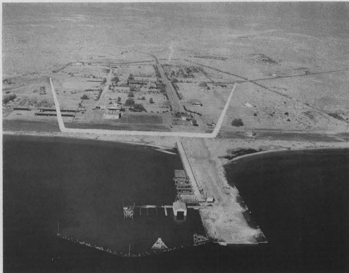
APPROXIMATE LOCATION of the dike now under construction at Salton Sea Test Base is shown in this photograph. When completed the wall will be 3,400
