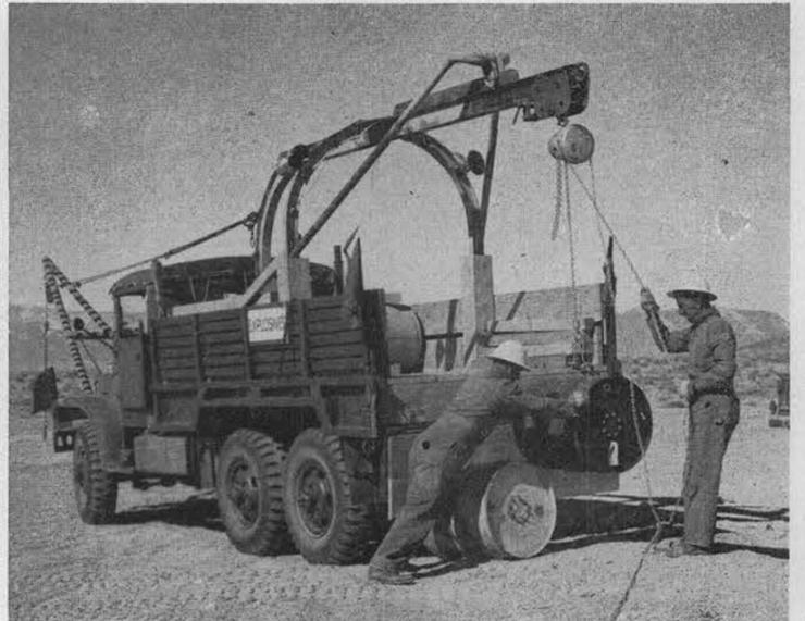
EXPLOSIVES—600 pounds of TNT in the form of an obsolete Naval depth charge are swung into position by Donadieu "Frenchie" Sonnier, 1932, as Jerry Ward, Field Test high explosives man, 5212, mans the hoist. The HE is detonated before a nuclear explosion to predict shock wave patterns.
