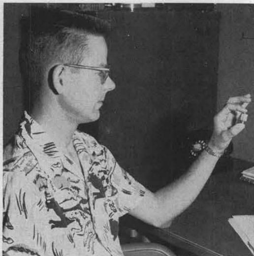
COBALT CONTAINER—Buzz Milton, supervisor of the X-ray Analysis Section, 1612-4, holds a small metal capsule like the one used to contain the radioactive cobalt isotope which makes relatively inexpensive radiography available to Sandia Lab.
