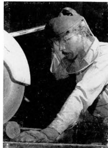
FACE SHIELD worn by Manuel G. Martinez, 2121, protects him from flying sparks and bits of sharp metal while sawing steel.
