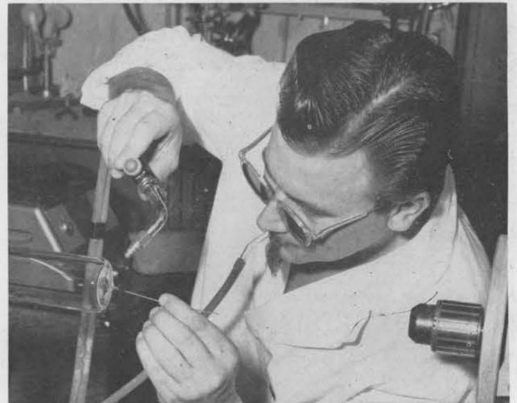
**DELICATE TOUCH** of Joe Chouinard, 1413, eases a wire filament into a vacuum tube being blown in the Physical Electronics Laboratory. Joe holds a flame torch to melt the glass and gently puffs through the tube to shape it into the desired form.
