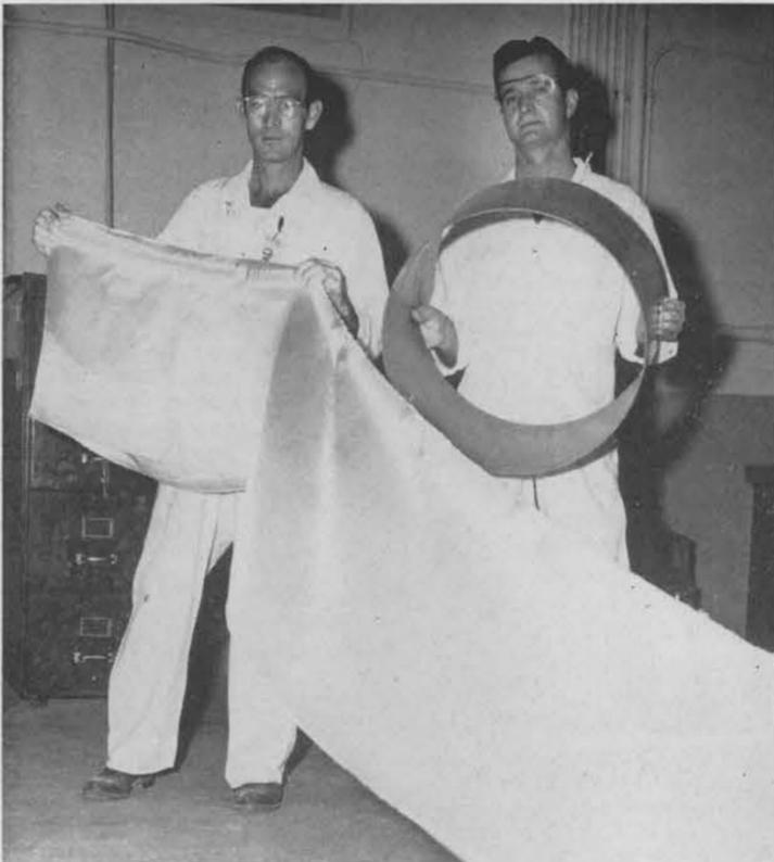
GLASS CLOTH held by Francis Pendergast is impregnated with resin and rolled on a mandrel to form a lightweight high-strength cylinder such as the one held by James South, right.
