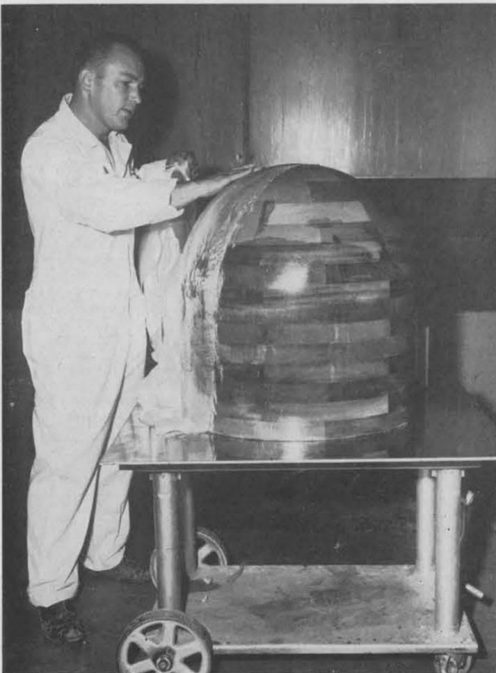
FABRICATION of dust cover for an outdoor camera is started here by Richard Olive. He is placing a layer of resin-impregnated glass cloth on a wood mold. He will build the layer to 1/8" thickness.
