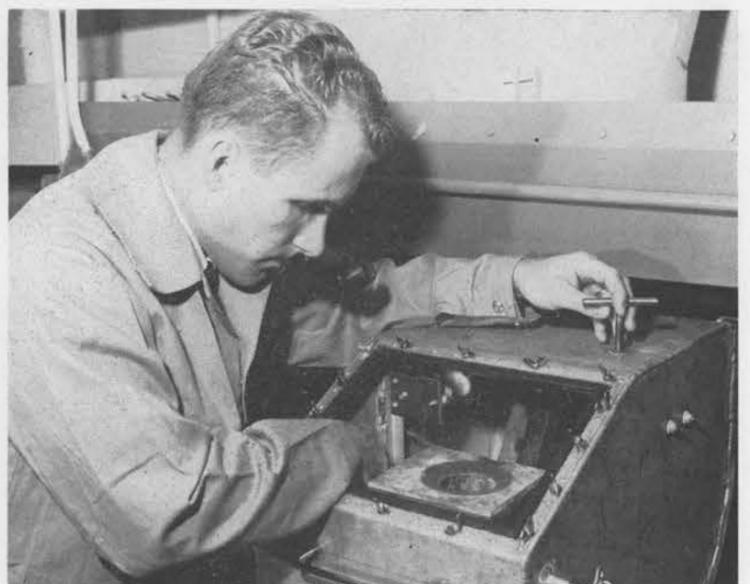
**CONTROLLED ATMOSPHERE** is often important in melting and pouring metals because elements in the atmosphere can combine with the metal and cause undesirable characteristics. Don Johnson, 1621-2, readies a special controlled atmosphere melting unit for use.
