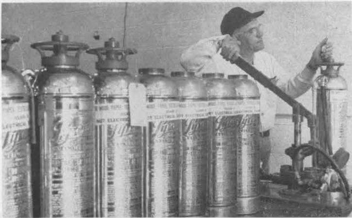
**EXERTING 350 lbs. pressure on a five-year-old fire extinguisher, a hydro-static test unit, operated by Jim Schenck (2415), determines if the extinguisher is in safe and efficient operating condition.**
