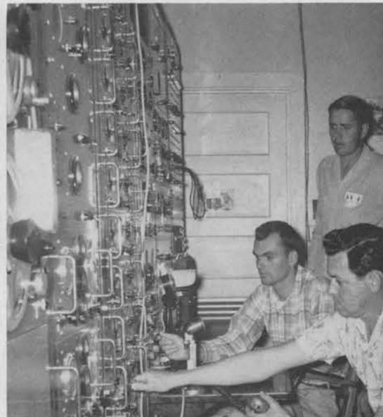
TELEMETERING CHECKOUT—Before the plane leaves Kirtland runway a complete checkout is made of telemetering equipment by (L to R) Wilbert R. Wood, Vernon M. Brewster and Clarence W. Young.
