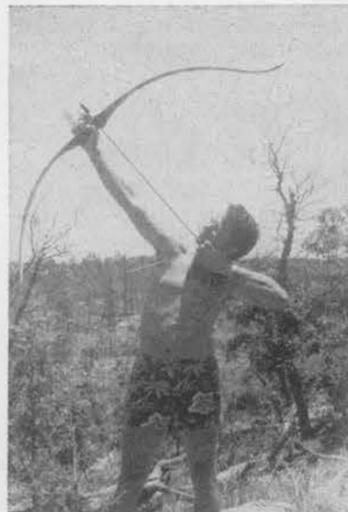
BOW AND ARROW was used by Gene Bussey to get a pulley line over some 125-ft. pines. With the line shot into position the rhombic antennas were pulled to the desired height.
