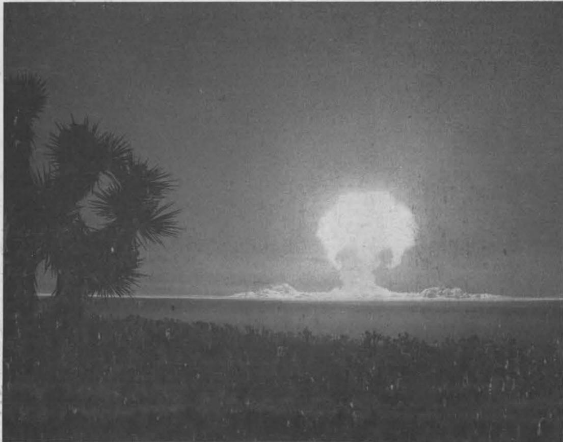
HOOD SHOT, of the current nuclear test series in Nevada, recorded the highest yield of any device ever fired in continental United States. The spectacular sight was recorded by a special camera built in Sandia Corporation's Optical Measurements Division. Bert R. Anderson operated the camera.
