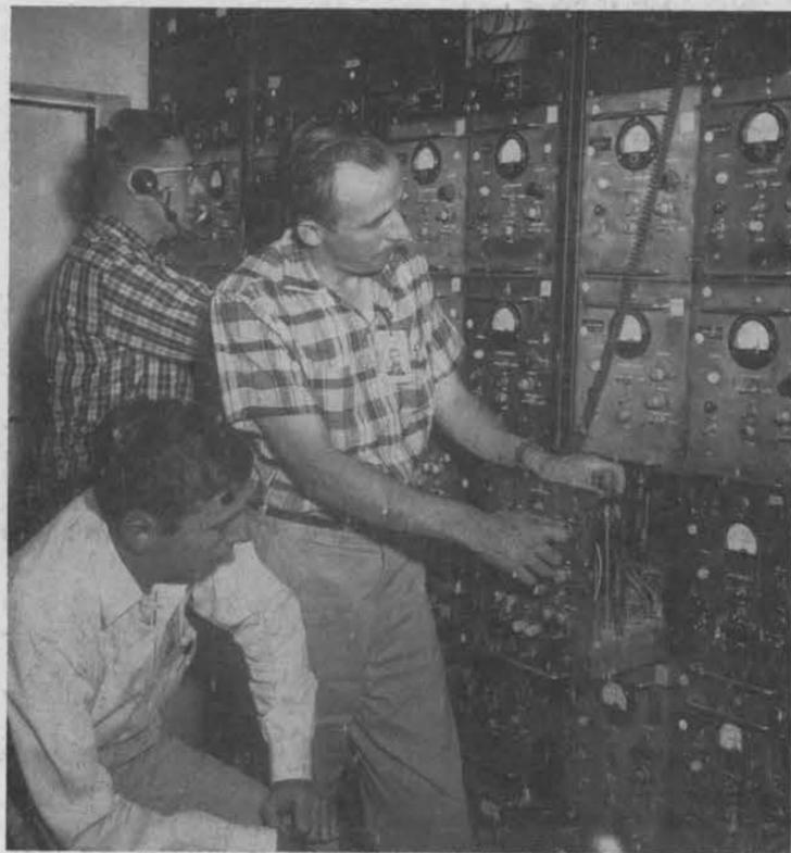
**DATA RECORDING SHELTER** at Coyote Canyon houses instruments that record blast effects. Jim Smith and Ed Vulcan (standing) with Jack Hughes (foreground) make adjustments on sensitivity recorders prior to an impending test shot.
