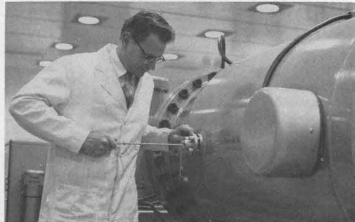
STEEL TANK, filled with carbon dioxide and nitrogen under high pressure, is checked by Herman Stein. The electric system enclosed in this tank permits a potential of more than two million volts.
