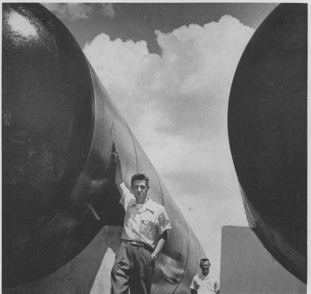
AIR STORAGE TANK for Sandia Corporation's wind tunnel facility (left) coupled to the present tank (right) together will store 5200 cubic feet of air to permit longer and more frequent tests in the wind tunnel. Demonstrating the site of the tank are Duane E. Randall (left) and S. S. Millwright.
