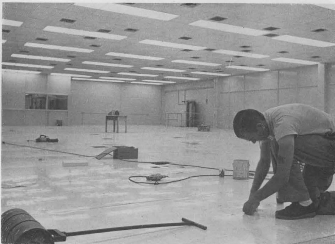
**NEARING COMPLETION** the special 705 computer construction worker. Removable floor panels allow room in Bldg. 880 receives final touches from a access to the electrical connection underneath.
