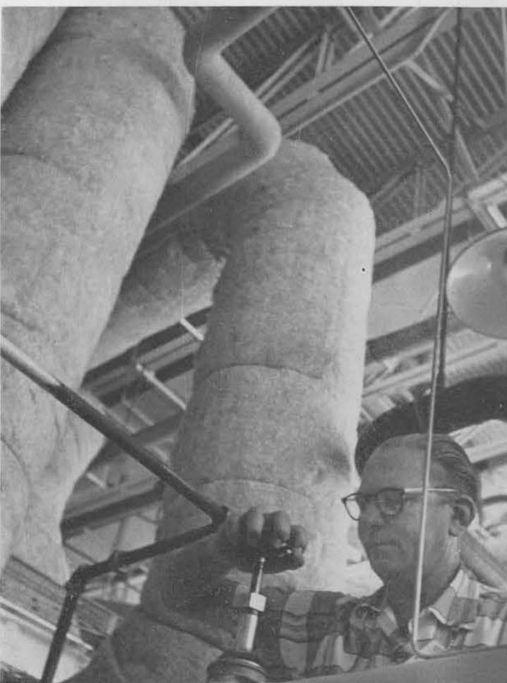
**AIR CONDITIONING** installation for the 705 EDPM facility is extensive. Vern L. Brockway (2411-2) makes final adjustments on the absorption refrigeration system of the cooling system.
