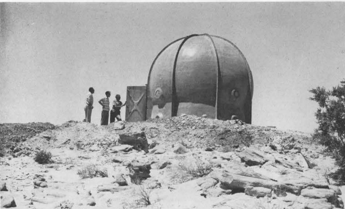
NEW RADOME to house weather radar antenna at Salton Sea Test Base is made of plastic which allows the unit to operate through it. Year around protection is given for the weather balloon track-
