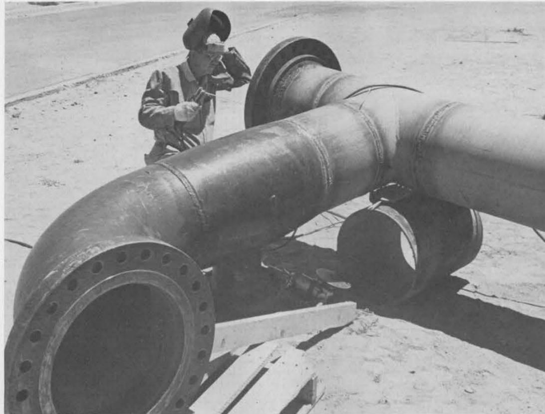
DRASTIC RESULTS are avoided with welds such as the one completed here by D. C. "Bob" Davis (2414). Proper welding is a must to withstand the tremendous 400 PSI Pressures of Wind Tunnel.
