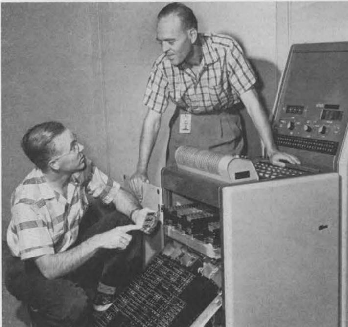
VERSATILE OPERATION of the "Blue Boy" Automatic Programmer and Recorder is made possible by these trays of interchangeable transistorized cards. Circuit arrangement of one of the cards is discussed by Robert Adams (L) and Clinton Purdue (both 1521).
