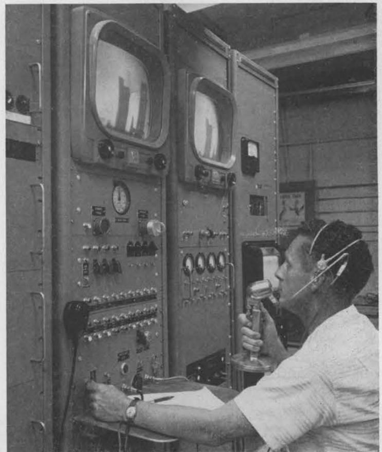
FIRING PANEL and control console for the rocket sled track is operated here by L. R. Myers (1613-4). On the TV monitor screen is a close-up of the Nike Booster rocket on a test stand near the track which was fired shortly after this photo was taken.
