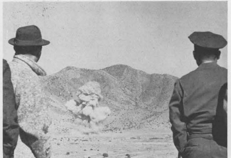
**MINIATURE MUSHROOM** blossoms as non-nuclear test shot is fired at Coyote Canyon. In preparation for the shot a pit 100 feet long was dug, the rocks removed, and the pit backfilled after pressure gauges were placed in a carefully arranged pattern. Results will show character of shockwave forces moving through the ground.
