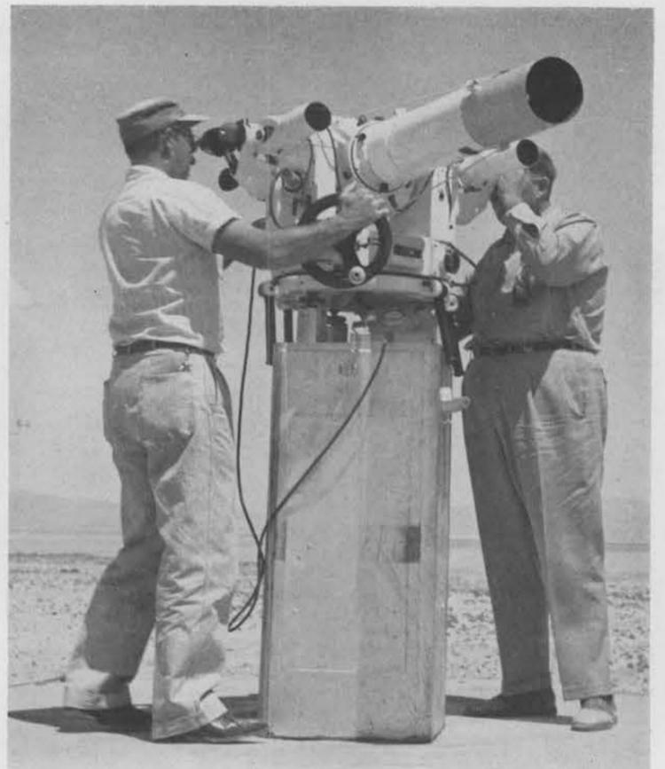
ASKANIA STATIONS at Salton Sea Test Base such as this one operated by Harvey Harter (5214), left, and Jim Keller (5225), will be used to calibrate meteorological equipment of the U. S. Weather Bureau and military services. This instrument is a photo cine-theodolite which records elevation, azimuth, and time of each frame of high speed film exposed during a drop test.
