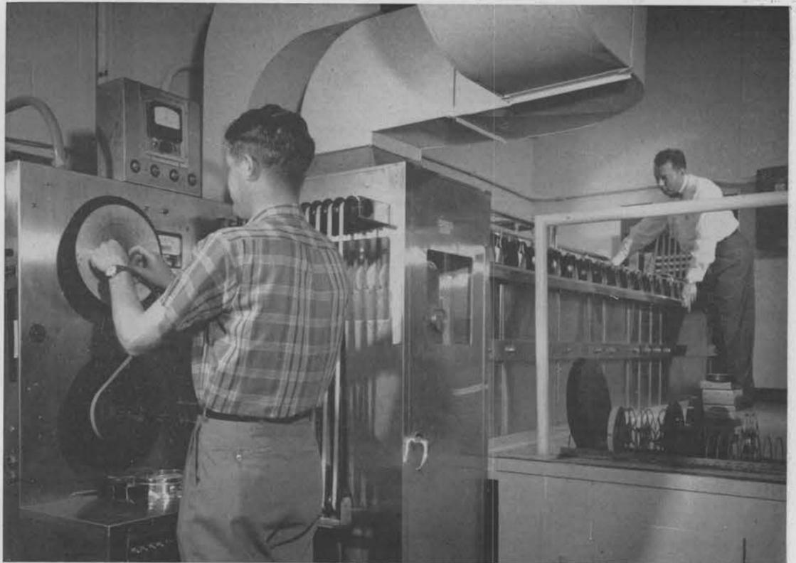
**NEW AUTOMATIC COLOR PROCESSING machine** of the Movie Division is operated by Wayne Hancock, left, while Jim Karo checks tension of the film moving through the tanks of the machine. Once controls are set for the machine, its operation is automatic as it processes 35 ft. of film a minute.
