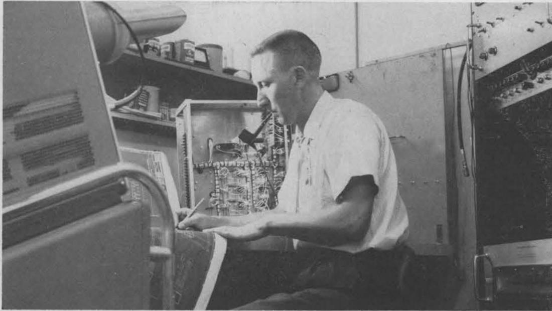
**POINT-TO-POINT** wiring check of production tester is performed by Bill Caldwell (2551-4). After complete check of the PT against the drawings, the tester will be given initial calibration.
