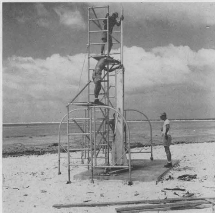
PRE-LAUNCHING CHECK is given one of Sandia's Chaff rockets used in attenuation studies of ORANGE and TEAK shots. Performing the circuit check are R. B. Allison (5143), on top, W. E. Walker (5143), next on ladder, and C. T. Force (5141), right. Hermann Wente (5141) is almost hidden by the rocket launcher base.
