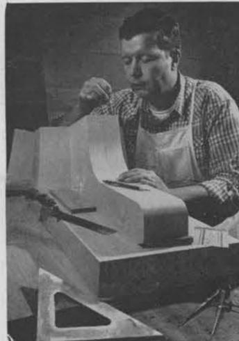
**CAREFULLY** marking wooden pattern is Thomas Mickey. The piece will be cast for a control mount for a tracking telescope.
