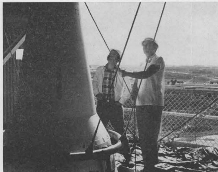
UMBILICAL WIRING from Sandia's telemetering package inside this Atlas nose cone is checked by Bill Arnold (5254), left, and Bob Pace (5254). The men are standing on the gantry platform.
