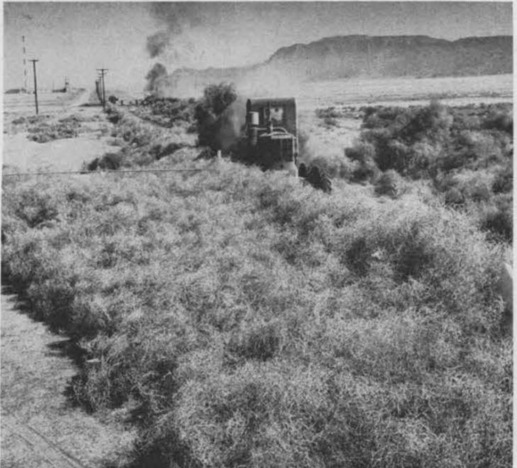
TUMBLEWEEDS OBLITERATE six ft. barbed wire fence in Area III. Grader pushes the weeds away from fence and piles them where they can be burned with a maximum amount of safety.
