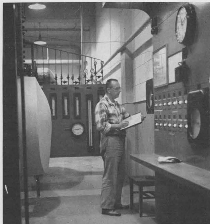
CONTROL BOARD for operation of steam turbine and chilled water refrigeration system, which cools Bldg. 802, requires close scrutiny by George W. McClure (4511). During summer months three shifts of men are required to keep system at top efficiency.
