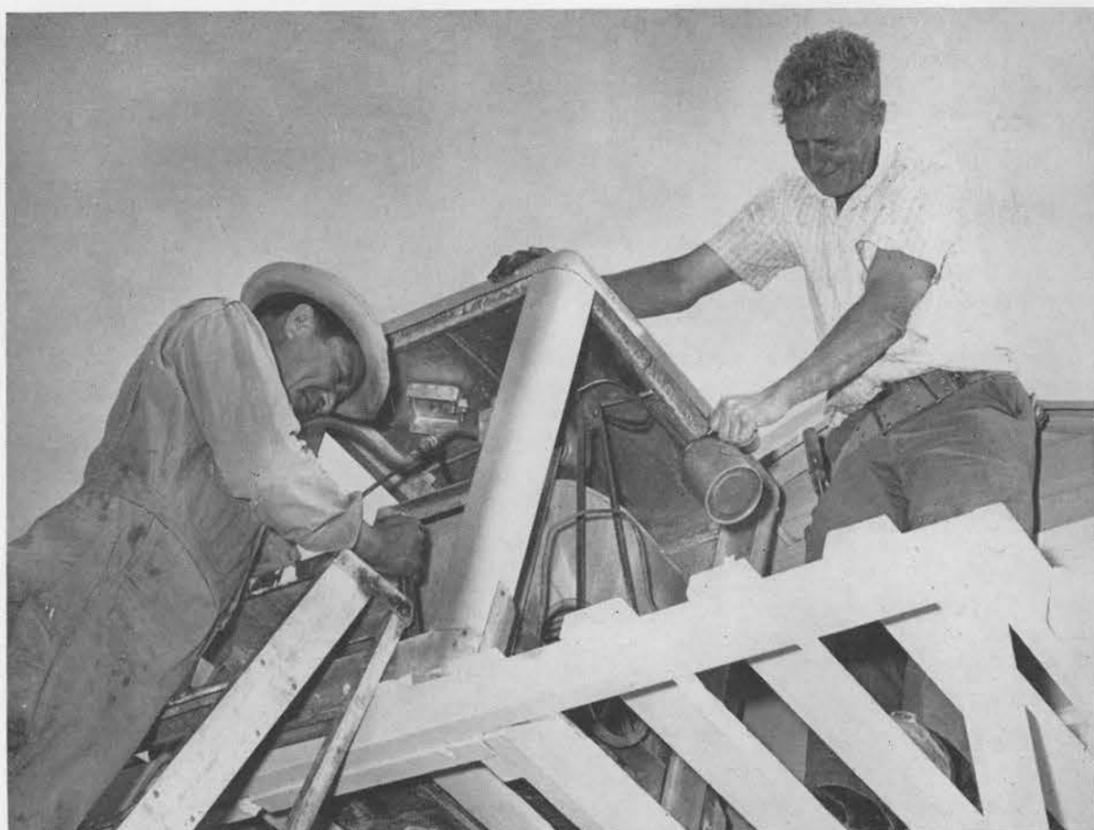
LUBRICATION and checking connections are necessary steps in yearly maintenance of evaporative coolers. Billie Rogers (left) and Charley Mills (both 4511) are readying this cooler for use on hot days.
