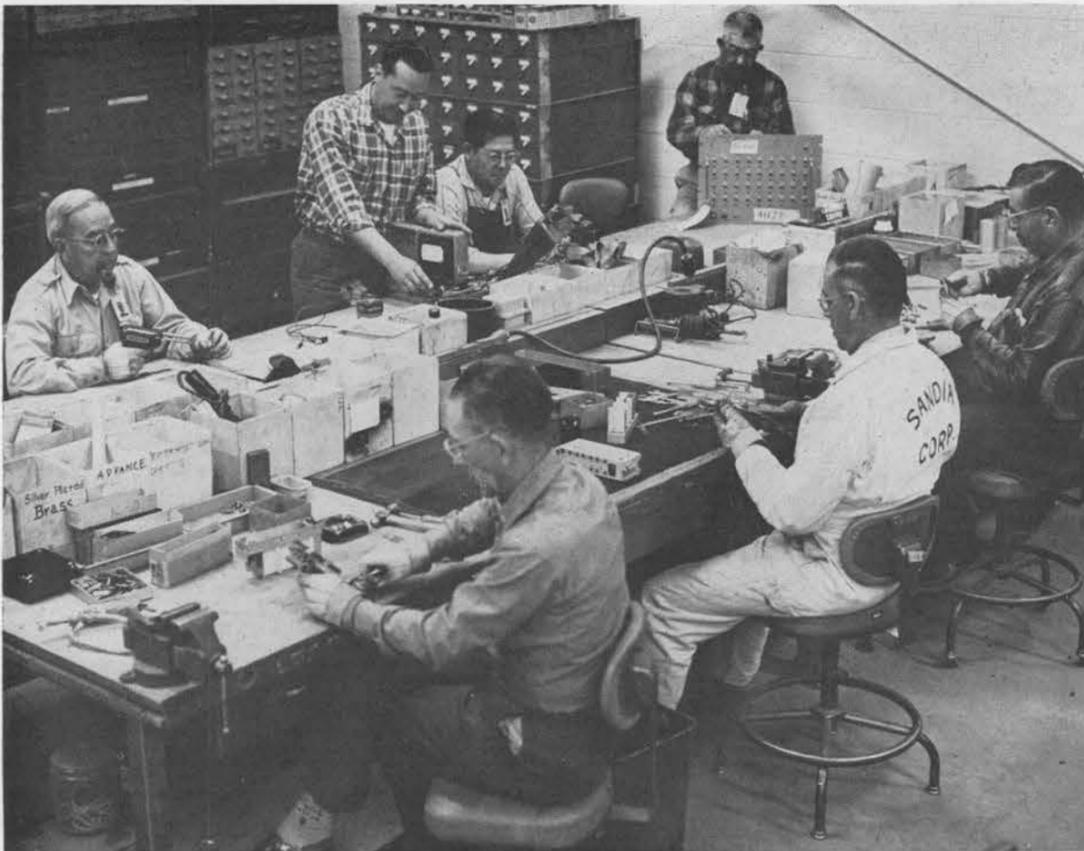
**DISMANTLING OPERATION** of used equipment to recover usable parts is performed by personnel of Processing Section 4621-2. In the background is a section of the extensive catalogued and stored supply of usable electronic parts maintained by the organization. Browsing for items encouraged.
