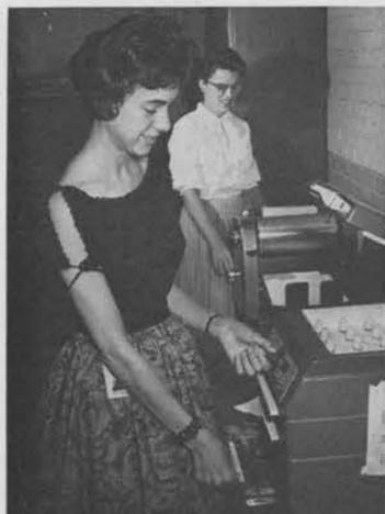
**SUSAN MAY** operates the Verifax Machine while Vanty Boley runs the Azograph machine in the back. Both processes help typists speed up work completion.
