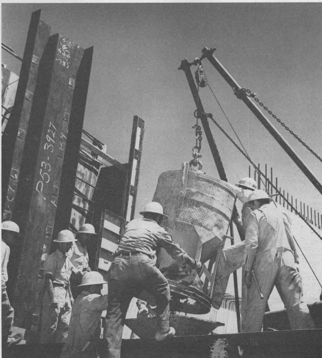
HIGH DENSITY CONCRETE was poured into reactor Facility last week. Doors, which weigh about 660,000 pounds, will be lifted by hydraulic power.
