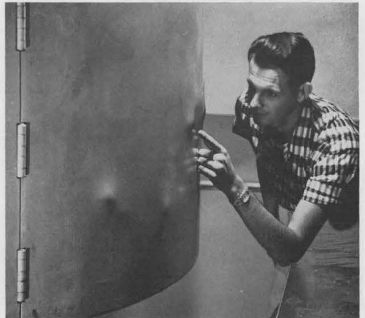
**FLYING PIECES** of a dummy component pounded these dents into the 1/4-inch steel protective plate surrounding the Livermore Laboratory centrifuge. Jack Workman (8121-1), centrifuge operator, examines the plate. The accident happened when the adhesive bond holding the component onto the centrifuge arm failed as the whirling arm reached a speed of 450 revolutions per minute.
