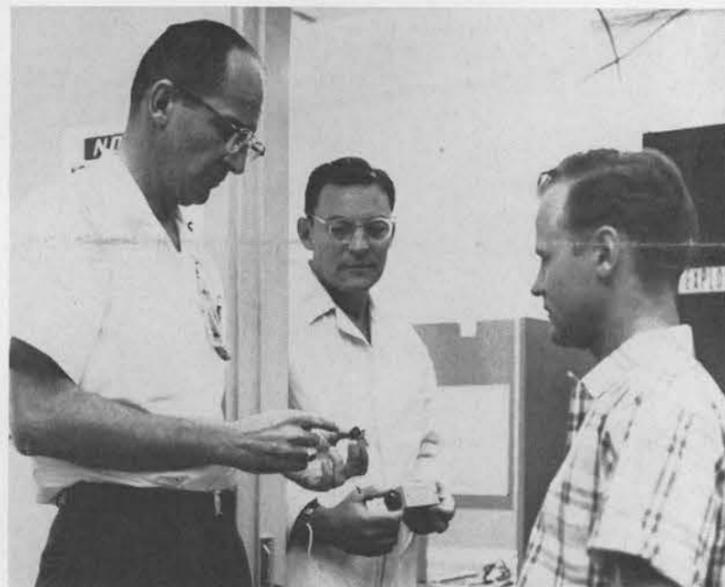
**IN STATIC-FREE AREA** located in Bldg. 809, safety engineer Verne Christy (3211), left, talks with Mel Ortega (1222), center, and Duane Stenberg about a fabrication problem in soldering wires to a connecting device for a small explosive switch. Ortega conducts the operation in the static-free area. Note the ground wire attached to his wrist, a safety precaution to prevent static.
