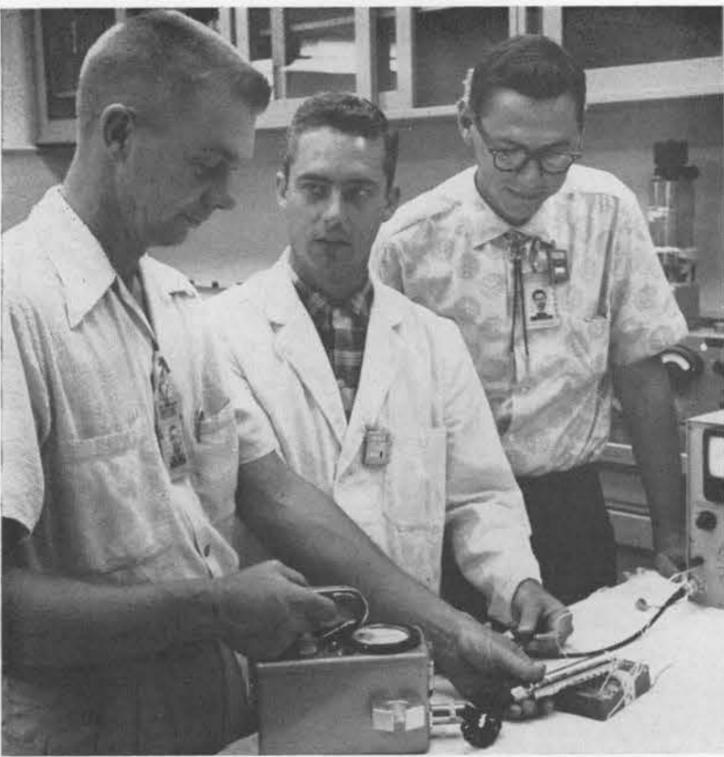
**MONITORING ACTIVITIES** include checking amount of radiation emitted from this nuclear cell battery which Ed Gooden (1631) is using. Milt Tucker reads the geiger counter while Harold Rarrick (right), section supervisor, watches.
