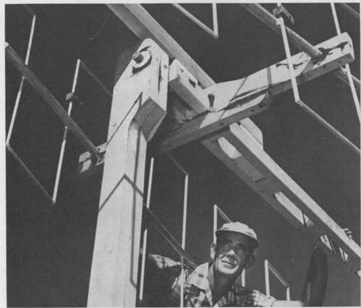
CONSTRUCTION DETAIL of the antenna support stand is shown above by Jess Denton. Only wooden pegs and glue (dark areas on wood) was used in the fabrication of the stand. Wooden axle rotates inside a nylon bearing for friction-free operation of stand.
