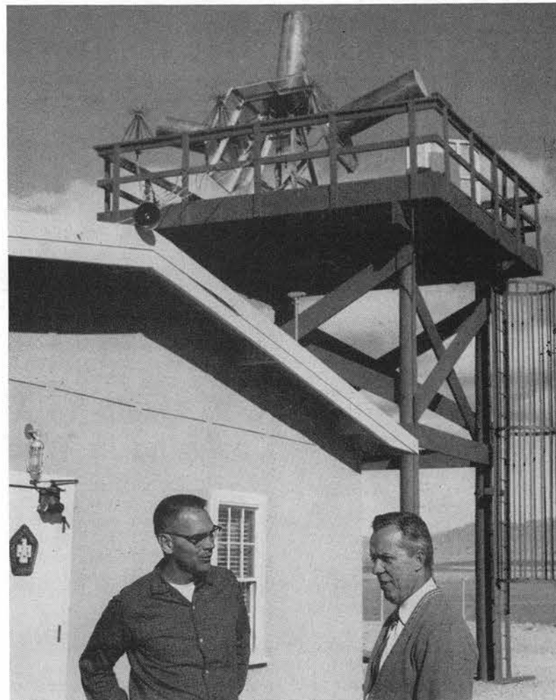
AT THE HEADQUARTERS and control building at Tonopah are (left) R. D. Statler, supervisor of Test Range Division 7212, and W. H. Everhart, supervisor of Tonopah Test Range Operations Section. Telemetry antennas are on the platform by the building.
