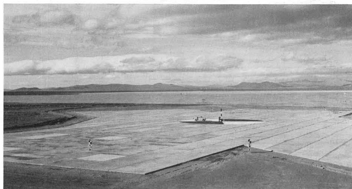
"X" MARKS THE SPOT for hard-target drops non-reinforced concrete, one foot thick. Each bar at the Tonopah Test Range. The target consists of of the "X" is 750 feet long and 220 feet wide.
