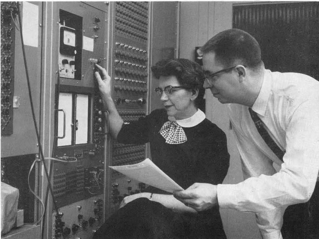
THERMALOG COMPUTER, designed to make heat transfer studies, is operated by Betty Brake, Plugboard to program problems is at left. Philip Class and other members of Section 7183-3.
