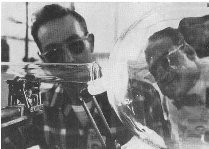
CAREFUL APPLICATION of the glassblower's art is required as Bert DuMars joins two glass pieces. The glass apparatus is a liquid nitrogen pump which will be mounted to an oil diffusion system.
