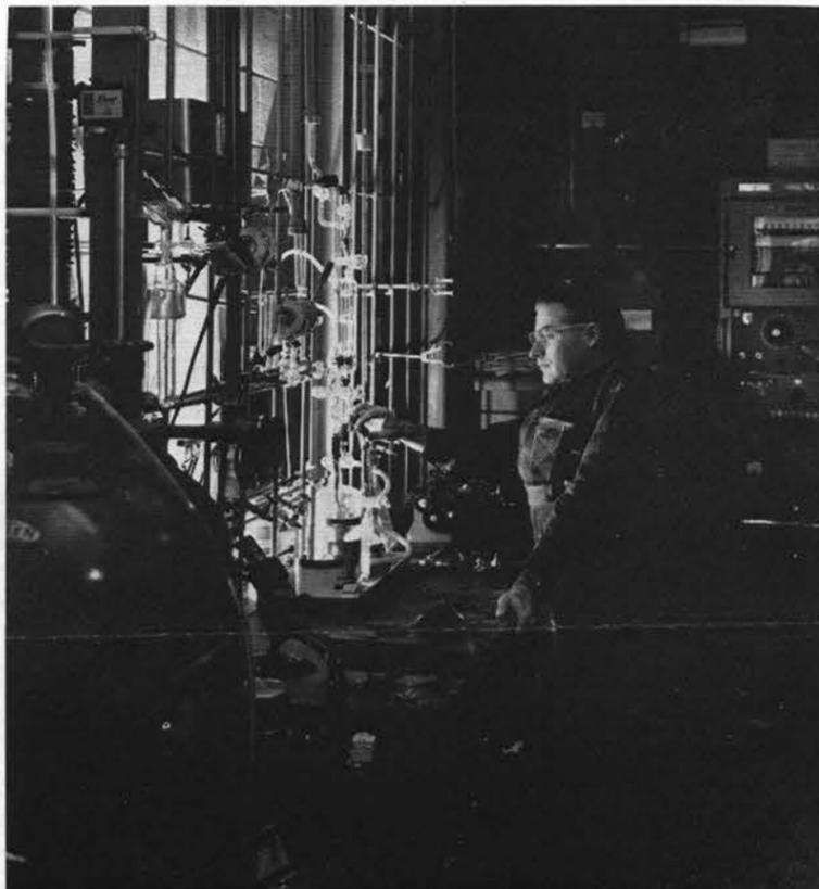
**HIGH VACUUM** system, recently completed at the Livermore Laboratory chemistry lab, is operated by Charles Arthur (8815-2). The system was designed to determine the hydrogen, nitrogen, and carbon contents of organic materials present in test samples.
