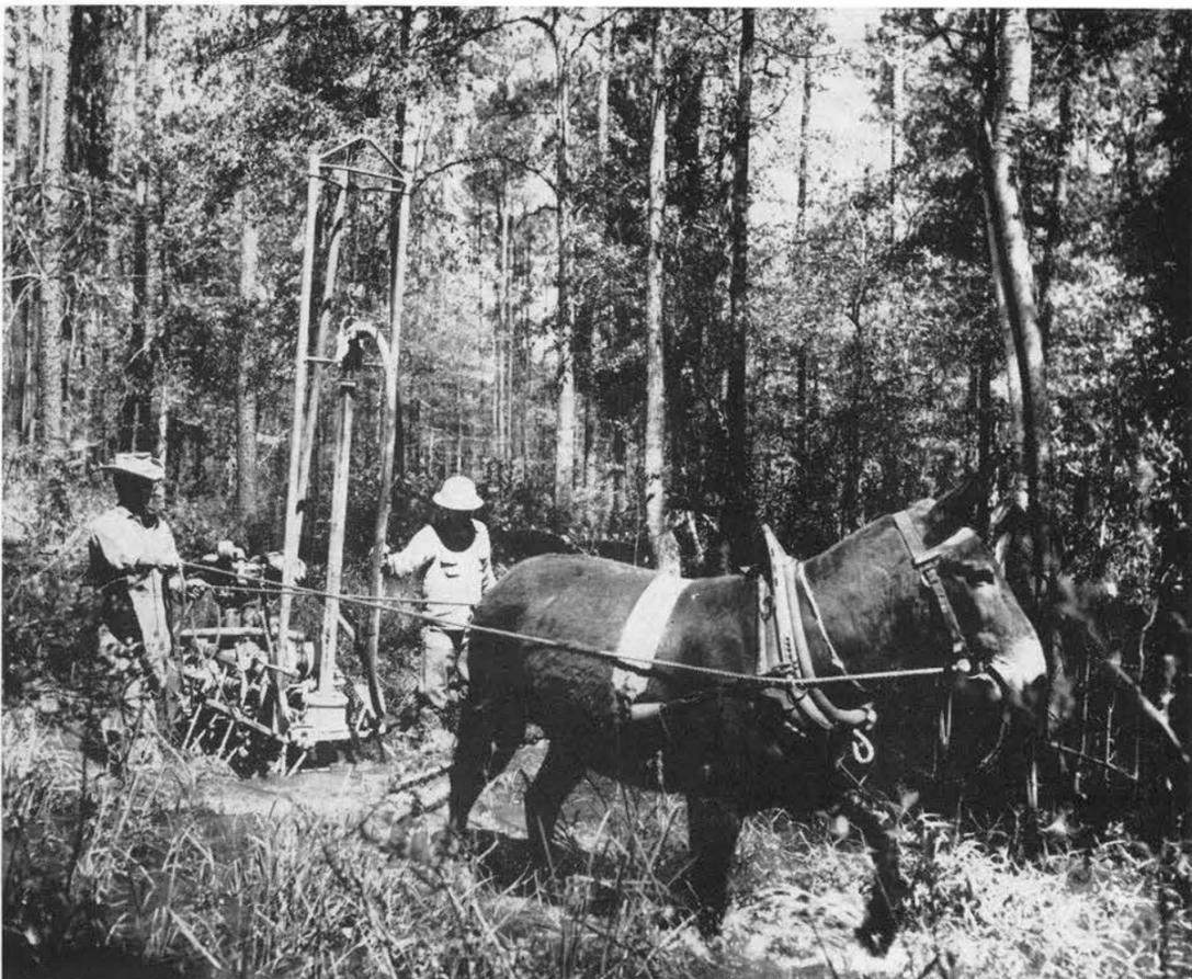
OLD FASHIONED MULE POWER proved to be the only feasible method of transporting a small drill rig through the swampland of Mississippi. The holes are being drilled in the Tatum salt dome.
