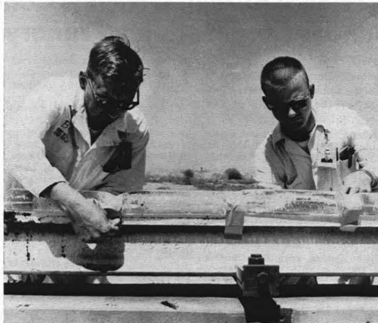
WATER FILLED polyethylene plastic bag, being filled by Dave Bickel, left, and Bill Kampfe, provides an effective brake to the monorail rocket sled which achieved a velocity of Mach 1.25.
