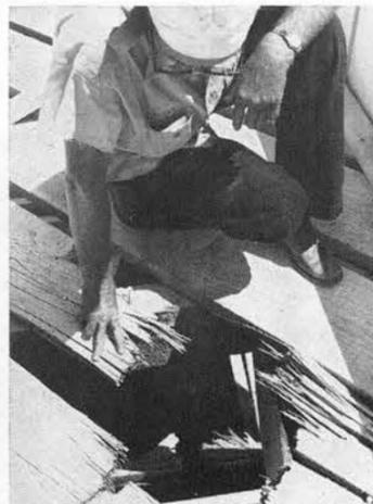
**HOLE CAUSED** by direct hit on water target by 500 lb. non-explosive bomb is examined by D. S. Cain. Instead of explosives, bombs carried electronic telemetering instruments. Drop tests were conducted almost every day, weather permitting.
