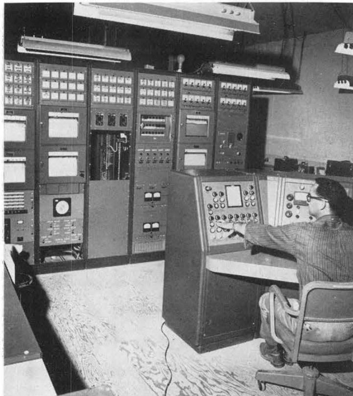
CONTROL CONSOLE for new reactor is operated here by Norman Lucas (5431). The instrumentation is a combination of commercial and Sandia-designed parts. Missing panel in center of photograph is at reactor site to check out the cooling system.
