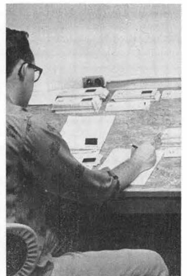
**IN FINAL STEP**, William Lewis gets 35mm IBM window cards ready to go to Copy Flow. The IBM cards will also be sent to microfilm banks located throughout Sandia Laboratory. At these locations, employees use printer-reader machines which magnify negative 15 times. Quick copies can be made of this size on printer-reader.
