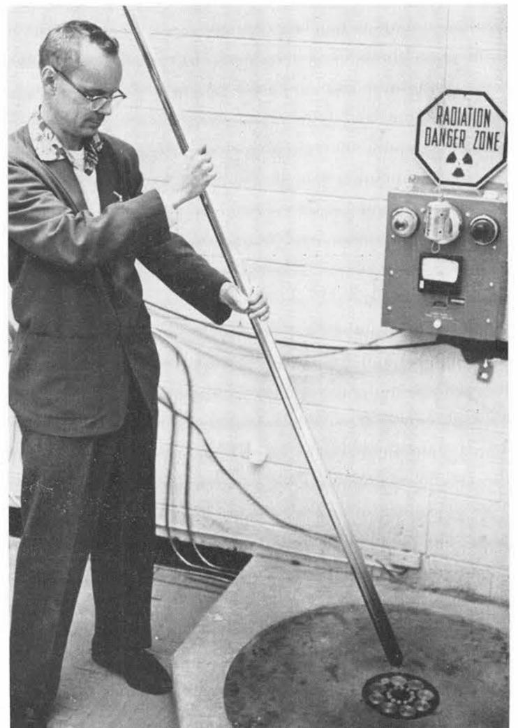
COBALT-60 SOURCE in Bldg. 802 is contained in concrete-shielded pit. Sample tubes, including six ft. Dewar tube held by Frank Truby (5151), may be inserted in center hole or in any of eight large circle areas in lower right corner of picture.
