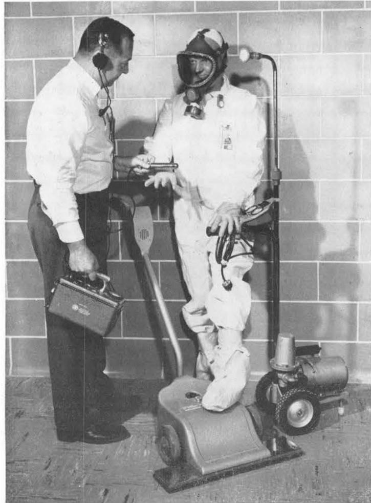
"TAKE ME TO YOUR METER," says Verne McNabney (right) as he and Bob Hanzel display radiation monitoring equipment used by the Health and Safety Section (8241-3) at Livermore Laboratory. New machine at right collects airborne radioactive and toxic particulates; machine under Verne's foot monitors alpha radiation on floor; and Bob holds conventional geiger counter. Verne wears protective equipment, including a respirator, in addition to a lapel air sampler, and a pocket dosimeter.
