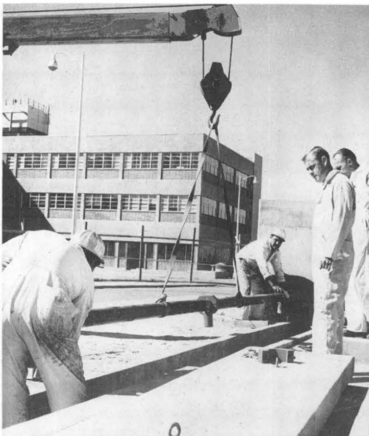
FIRST SECTION of the 80-ft. barrel of the new helium gun is positioned in a trench between two underground rooms. Millwrights are Sam Tabet and Manuel Lucero of Section 4512-1. Right are Sig Thunborg, Jr., and Earle Anderson (both 5134-1).
