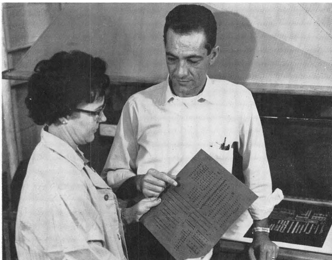
**NEW PHOTSENSITIZING** technique for numbering circuit boards, discussed here by Don Tassano, right, and Jessie Berry, both of 8223-3, requires only one man-hour for entire process. Negative used to expose numbers on plate is shown in this photo on the light table behind Don.
