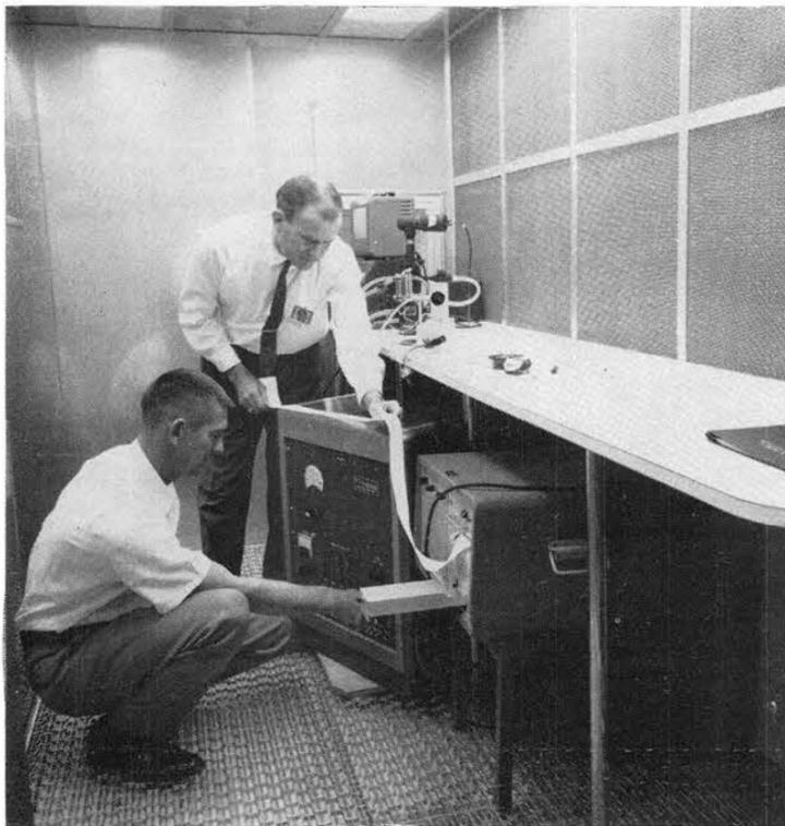
DUST COUNT DATA showing the extremely low level of contamination in Sandia's new ultra-clean room are taken by W. E. "Bill" Neitzel (left) and Willis J. Whitfield (both 2564-2). Super clean air enters the room through the bank of absolute filters over the work bench at right, and sweeps dust particles away from the work area and into filters located beneath the floor grating.
