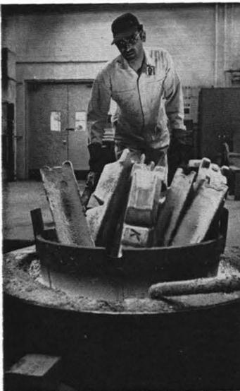
"CHARGING" the furnace, Damacio Sandoval watches aluminum ingots slowly sink into a white-hot gleaming mass. Giant crucible holds 900 lbs. of casting metal.
