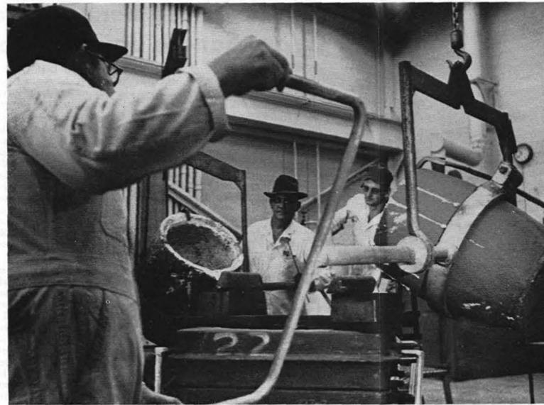
SMOOTH TEAM WORK is exhibited by Foundrymen during large pour. Inside the mold will form a 1000-lb. section of Sandia's new wind tunnel facility. Constant rate of flow into the mold is maintained up to 20 minutes until pour is complete. Foundry produces extra-dense aluminum.
