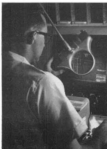
INSPECTION AND MOUNTING of microfilm in aperture card is completed by William F. Lewis (3444-3), operating a semi-automatic mounter. Before mounting film, he checks its drawing number, issue, and security classification against data on card.
