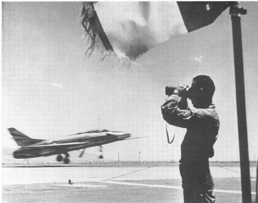
AIR NATIONAL GUARD F-100 streaks in for a landing at Kirtland. Ken Sarason checks returning planes as they approach to make sure landing gear is down. The "buddy system" helps avoid possible landing mishap.
